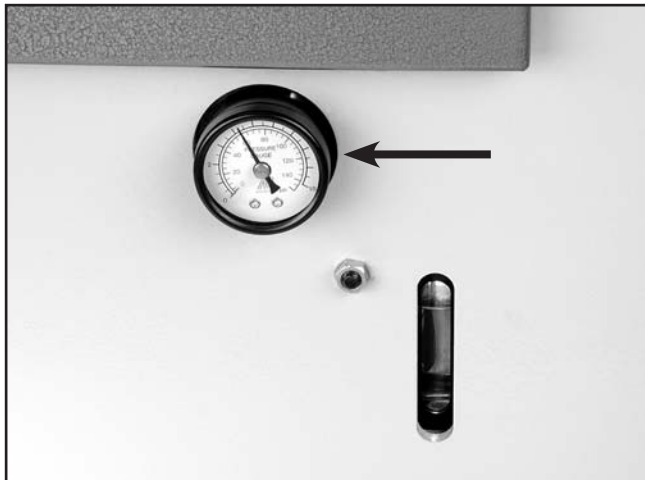
Figure 17. Air pressure regulated to 60 PSI at the gauge located on the outside of the cabinet.
